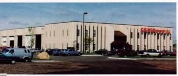
INDUSTRIAL/WAREHOUSE FACILITIES: C. S. McCrossan Service Facility, Maple Grove — Precast wall panels, beams, columns, double tee roof and Spancrete floor.
