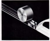
Remove paper and install 4" wide EPDM strips over tape, hand roll all bonded surfaces.
