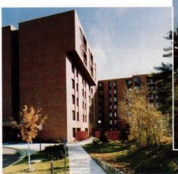
**HOUSING:** Robbins Landing, Robbinsdale — Prefabricated concrete walls, Spancrete floors and roof.
