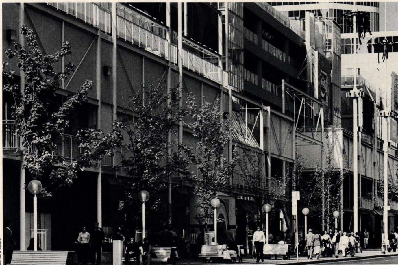
The facade of the Centre's outer "edge" on Yonge Street is a light steel framework hung by tension cables—"reminiscent of the North American cast iron period." Glass-roofed "Galleria" (opposite) soars 127 feet from lowest level.
