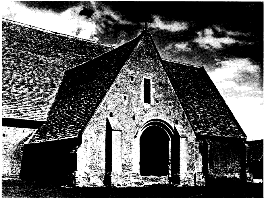
West porch is so admirably proportioned as to seem an organic appendage of the main building. Light is admitted to interior through vertical slit window and, on all walls of the barn, by put-log holes left by stonemasons' scaffolds. Transverse section of the west porch (below) depicts the timber framing system as essentially the same as that in the main structure. Oak elbow beams are from trees trained to yield such structural members.
