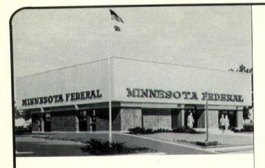
Minnesota Federal Savings & Loan, St. Cloud, by Voigt & Fourre, Architects, features stucco embossed steel wall-panels applied over structural steel framework.
