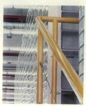
Composition of ordin nary materials assumes t quality of sculpture. Minimal pipe railings are mented by the simple security details—pla cized wire lines runs augest of astining between vertical po-made taut by the kir sts and d of y used ctric turnbuckle common on a clothesline. Ele wiring that wends fr om fixture to fixture visual y undulates, as if set in r notion by ceiling fan.
