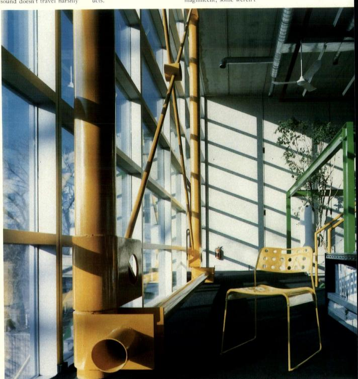
olychromatic scheme en-ches industrial details verywhere: Blue steel off-ie-shelf plates for steps re topped with black rub-er treads which are opped short of plate's dge to stress a veneer haracter. Structural steel onnection shown here ainted in "IKOY Green" ilstrates firm's design trategy: "Some firms weld bolt. We do both for lear design expression." right yellow flange as embly anchors wind races (opposite).
