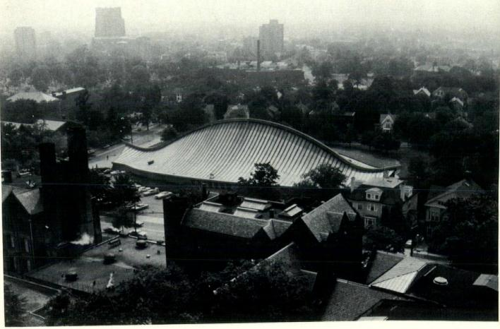
NEW HAVEN, CT—Four steel cables suspended from a center concrete arch give the intricate 5,500-square foot roof of Yale University's David S. Ingalls Hockey Rink the appearance of a colossal whale swimming across the campus.
