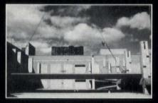
lifting the 50,000 pound precast, prestressed double Ts over the top of the existing five-story building and lowering them into position. This was accomplished with precision teamwork and 2-way radios.
