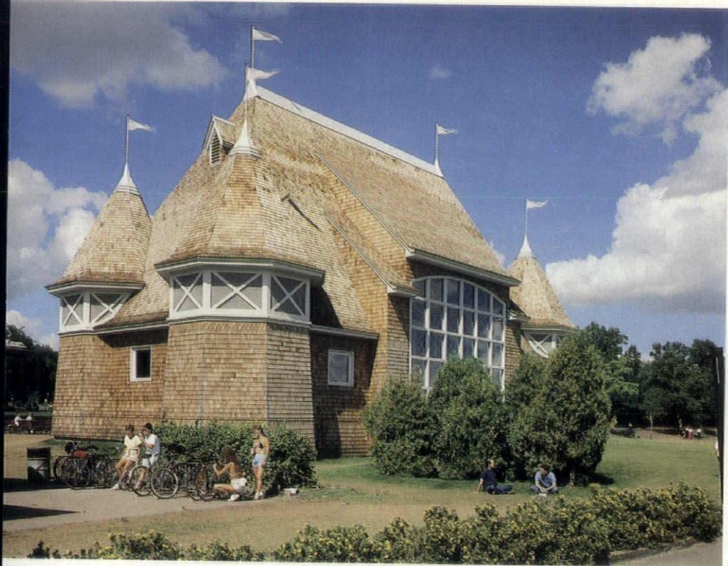
The shingle style design recalls a more romantic architecture popular in the late 19th century (left). But romanticism is fledged with functionalism. The base of the turrets and wings, in addition to providing storage for musical equipment, contains a ramp that enables accessibility for handicapped musicians.
