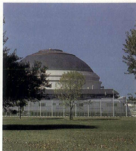
The 96-foot diameter of the Crown Space Center dome would fit comfortably inside the Pantheon. The segmented steel frame has sixteen radial ribs connected by horizontal tie beams. The space between the ribs is spanned by lightweight concrete sprayed onto pie-shaped sections of heavy pre-formed metal lath.
