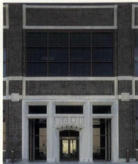
One of the building's more striking features: ornate limestone-framed entrances (above). Ankeny Kell kept the stonework for the two original entrances but designed modern glass doors that are recessed behind the limestone frames. Thus history is respected and convenience served.
