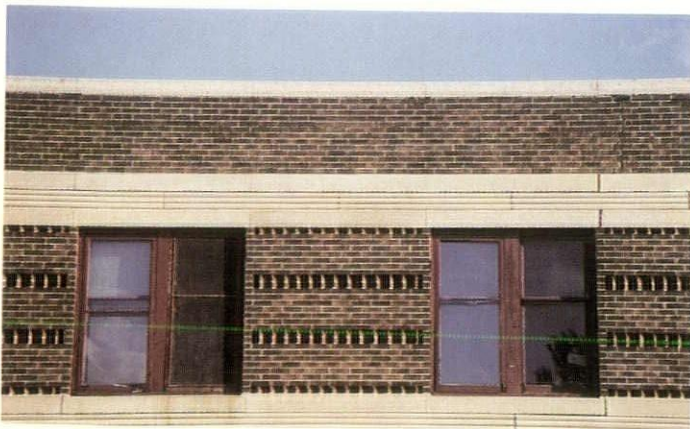
Serrated soldier courses create powerfully textured horizontals on a modest commercial block (above). Meticulous care in design and detailing, the use of two brick colors and special brick shapes enhance the Herman Miller showroom by Meyer, Scherer and Rockcastle (below).
