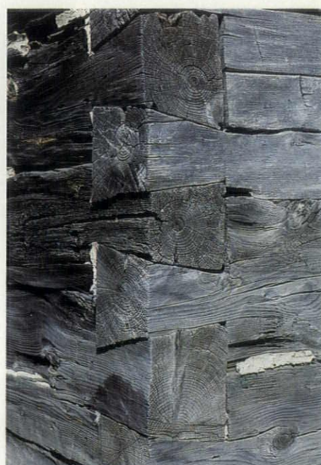
To craft their sturdy buildings, Finnish carpenters used several methods of corner timbering. Here, from left to right, a saddle-notched joint on the Pyhala horse barn; double-notched joinery on the Nelimark sauna; and a fully dovetailed corner joint on the Hebl house.
