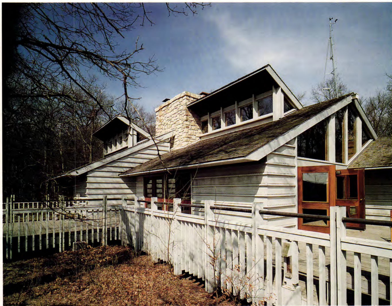
The center is oriented toward the sun. A three-sided deck and clerestory windows (above) open to the outdoors, while the broken-gabled form reduces the massing, allowing the building to slip unobtrusively into the setting.
