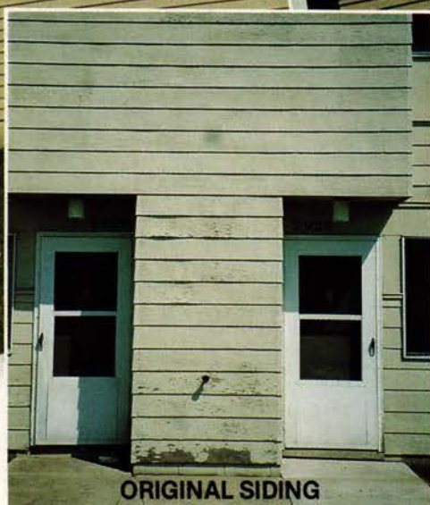
Siding Failure is obvious in this entryway photo.
