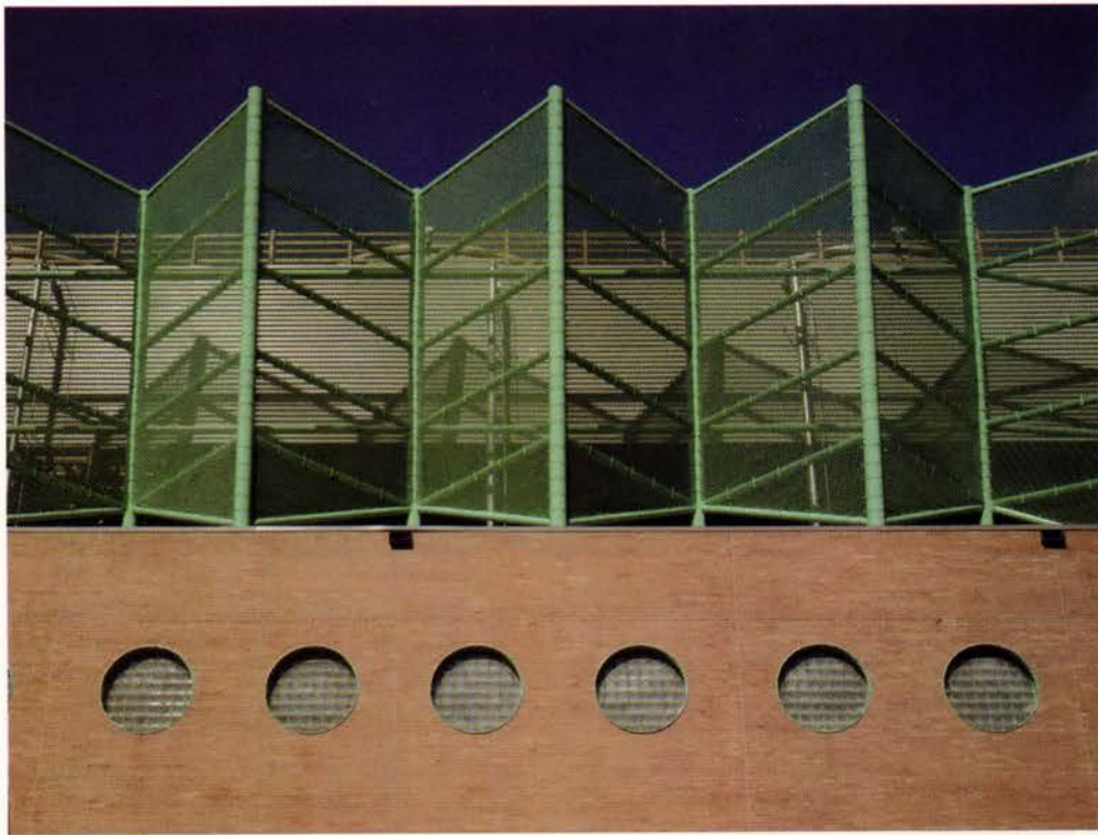
The green, sawtooth-patterned crown (left) hides the rooftop cooling towers. The facility is raised one level above grade (plan below) to allow for street-level parking. The interior is all mechanical and laid out on a rectangular plan.
