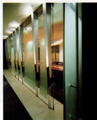
A metal-framed glass wall divides the conference room from the lobby (above and opposite). The wall, highlighted with sand-blasted glass panels, filters light into the conference room (left). Contrasting wood tones add warmth to the lobby (top).
