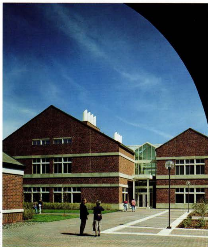
The Ardolf Science Center offers a traditional architectural presence (above and below) on the St. Benedict campus, reinforcing an emerging quadrangle. The interior is strikingly minimal. A granite stairway with stainless-steel railings (opposite) leads to the second level, highlighted by a glass-block floor (right).
