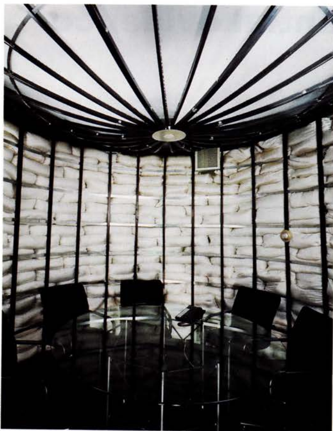
The circular conference room (above) is a wood-and-metal grid surrounded by sandbags and a suspension-cable grid holding the bags in place. A 200-foot metal undulating wall (opposite) punched with holes divides the space. The U-shaped floor plan (below) places services spaces, editing rooms and such toward the middle and work spaces behind the outer undulating wall.
