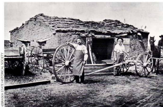
A sod blacksmith shop in West Union, Nebraska featured a lapped-sod roof (above). The McCone sod house (opposite) is a reconstruction of an 1880s "rich-man's" soddy near Sanborn, Minn., which is a museum and bed-and-breakfast.
