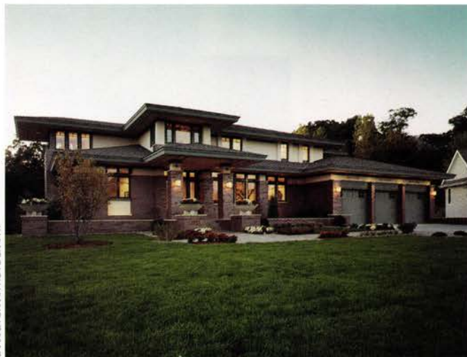
SKD Architects used computer images (top) to refine massing, roof projections, placement of exterior lighting and brick color. The architects eliminated a circular brick wall and added brick banding and battens under the overhangs as a result of this study (above).
