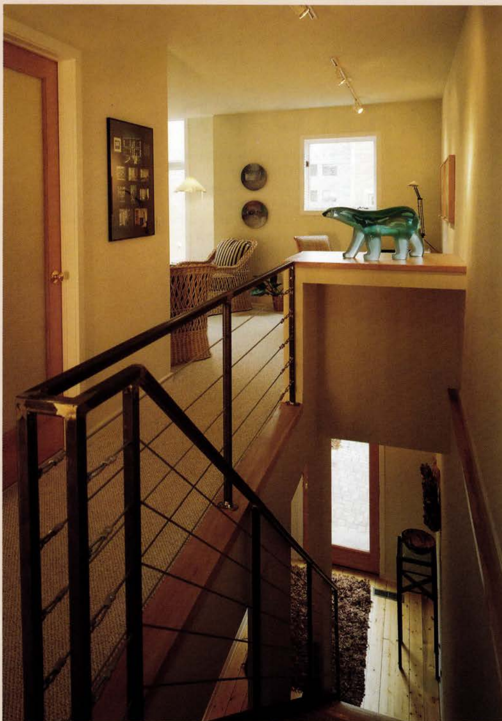
Steel staircases with maple treads and taut cables are standard features in each unit.
