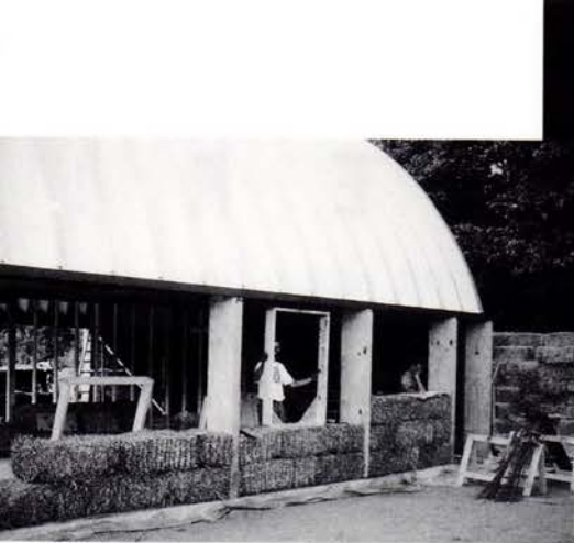
Corbin and Geisen also built a workshop on their property using the same straw-bale construction as their house. The building is finished in wood and stucco siding and a metal roof.
