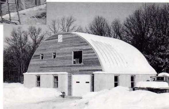
Corbin and Geisen also built a workshop on their property using the same straw-bale construction as their house. The building is finished in wood and stucco siding and a metal roof.
