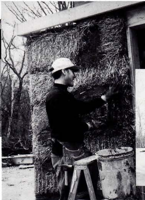
A truck hauls in bales of straw (below) to be used for Laura Corbin and Ken Geisen's house. Construction involves post-and-timber framing (above), piling up the straw insulation (center), and finally adding traditional exterior stucco siding (right) and interior lime-plaster walls.
