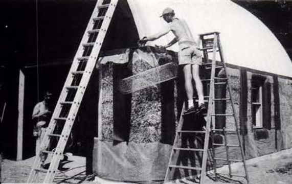
Corbin and Geisen also built a workshop on their property using the same straw-bale construction as their house. The building is finished in wood and stucco siding and a metal roof.
