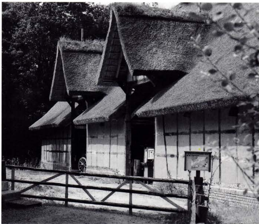
Post-and-beam construction with wattle and daub, Kommern, Germany.
