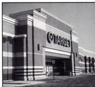
The Target Store in Stillwater, Minnesota, illustrates the smart look of 4" high decorative rock face CMU's complemented by 4" and 8" high Ground Stone Masonry Units to provide the ideal combination of strength, aesthetics and economy.
