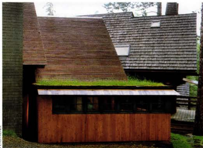
Sod roof on the Brandenburg Studio, designed by David Salmela
