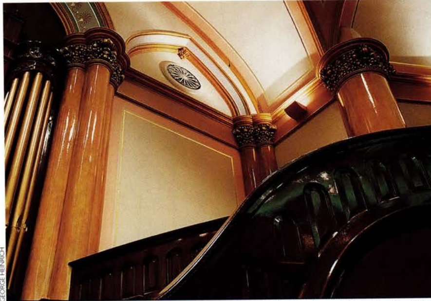
The color package for the sanctuary included a rose-colored band bordered with gold leaf on either side of plaster groins and a gold glaze on columns (above left and right). Collins redesigned the choir loft (after restoration, opposite above; before restoration, opposite below) to better connect the upper and lower areas of the sanctuary.
