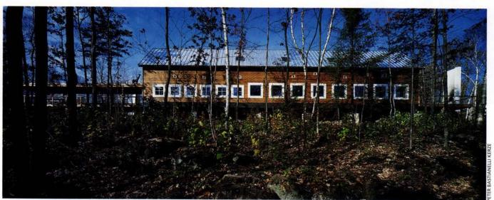
the area's boathouses and fishing shacks. He specified a galvanized-metal standing-seam roof (a nod to the corrugated-metal roofing favored for fishing shacks); left the exterior of the dining room unfinished (in homage to the vernacular tradition of leaving siding unpainted); and had the exterior siding on the kitchen and service wing painted "almost black" (to mimic tarpaper sheds).
