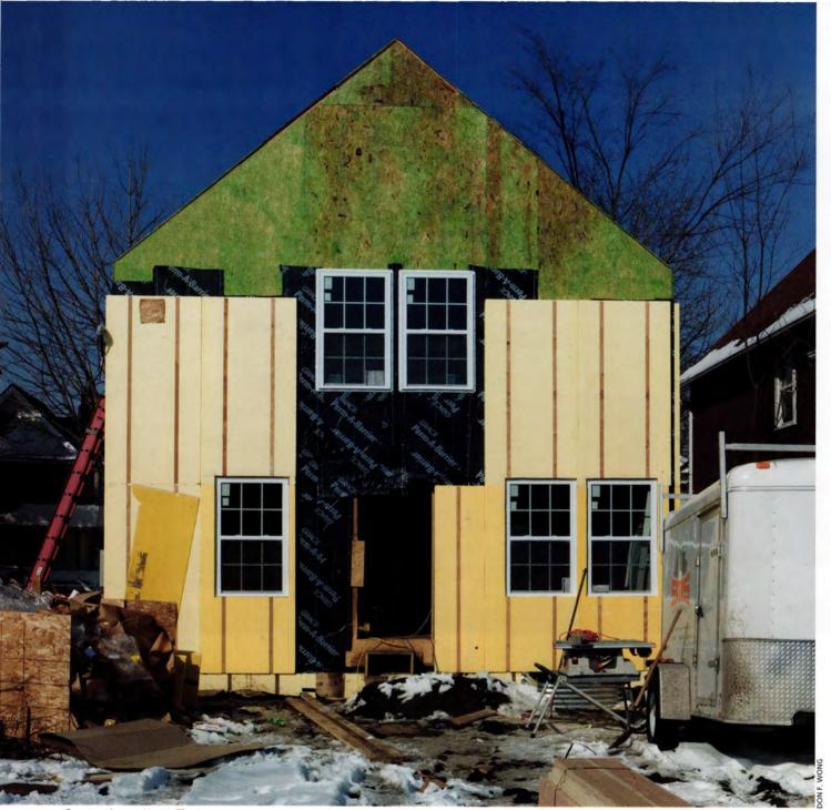
Construction on House Three, now nearing completion, reveals the layering of the wall system: OSB panels, waterproof membrane (black), and Styrofoam insulation (yellow).
