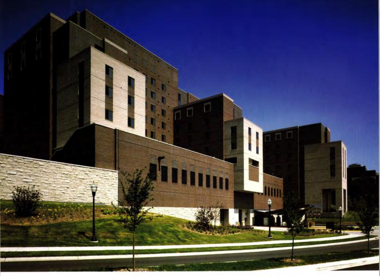
PROJECT South Mall, Riverbentl Commons, University of Minnesota LOCATION Minneapolis, Minnesota ARCHITECT Ellerbe Becket, Inc. MASON CONTRACTOR Gresser Concrete/Masonry FIELD BRICK (dark) Three blends of Sioux City Brick nationally recognized natural ironspot velour modulars. (Available in Modular, Norman and Utility)
