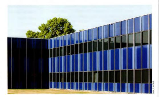
Right: The two-tone bright-blue panels set in brushed aluminum mullions create thin, vibrant, and visually textured curtain walls. Opposite: When completed in 1958, the original nine pavilions housed 500,000 square feet of office and manufacturing space.
