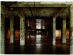
Inside the mill museum, parts of the original structure, including wood beams in the exhibit area (above) and the steel-truss structure in the rail corridor (opposite), were incorporated into the renovation. In the lobby (left) new square concrete columns are interspersed with the old round ones to open up the spacing, and the pattern for the wood ceiling scrim was created by scattering wheat berries on a copier and blowing them up to size.
