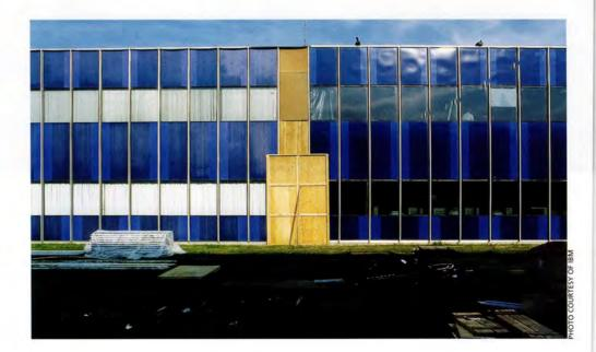
Right: In 1980, IBM replaced all of the original curtain-wall panels (left side) with identical new ones (right). Opposite: By the early 1980s, the campus had expanded to 24 pavilions spanning two million square feet.
