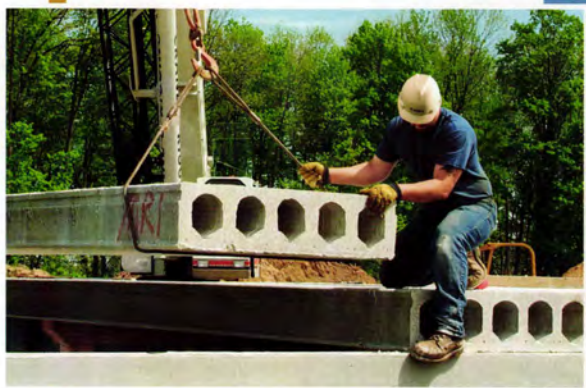
This photo illustrates the installation of hollowcore plank. County Materials' hollowcore plank saves on time and manpower, offering an easy alternative to pour-in-place for multi-unit structures.
