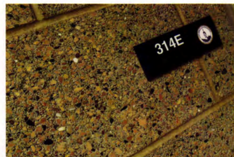
The arts addition includes more than 45,000 units of Ultra® Burnished decorative concrete masonry units in the Autumn Oakleaf color mixture.
