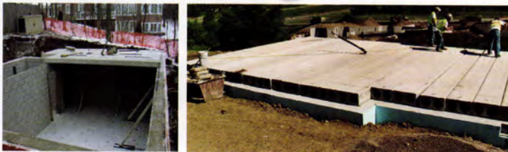
Photos of Molin Concrete hollow core planking being installed on a home
