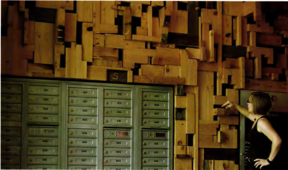
Salvaged Douglas fir cut-offs / Wood Wall by Souliyah Keobounpheng / Silvercocoon Design, Mpls, MN
