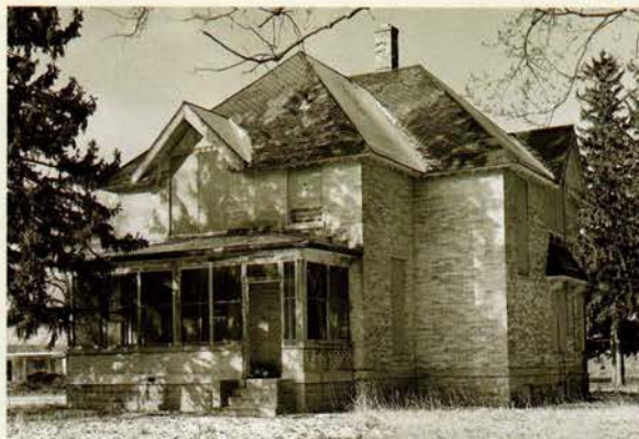
#152: OFFICER'S QUARTERS The building was mothballed in summer 2008. It was also re-roofed, and portions of the eroding roof structure were replaced.
