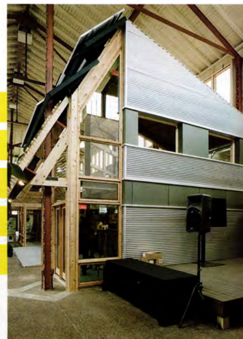
This project changed the way the SALA team thinks about green roofs. Here, solar panels work in concert with a terraced slatting system to heat and cool the home.
