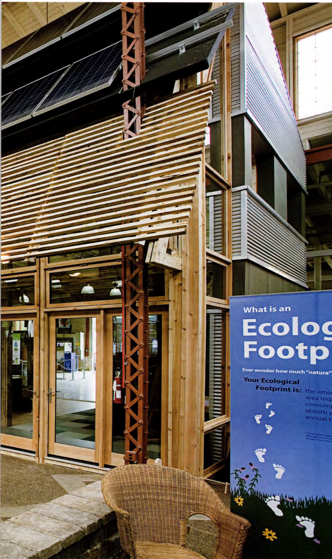
This project changed the way the SALA team thinks about green roofs. Here, solar panels work in concert with a terraced slatting system to heat and cool the home.
