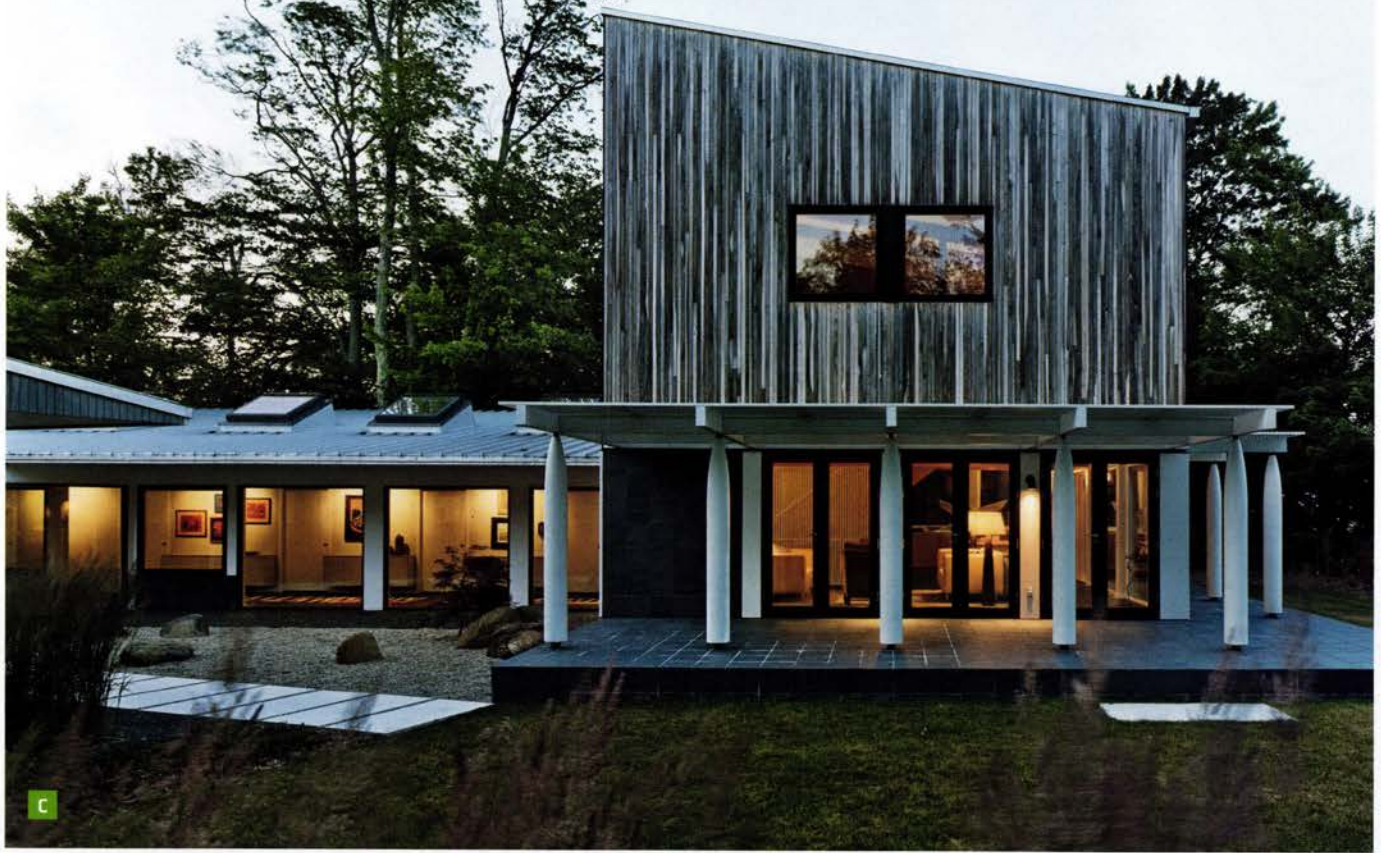
The main living spaces occupy a two-story structure (C), with a terrace and colonnade extending the living and dining activities outside. The living room (E), with the master bedroom mezzanine above it, overlooks Lake Michigan on one side and the house's secluded, contemplative garden (D) on the other.
