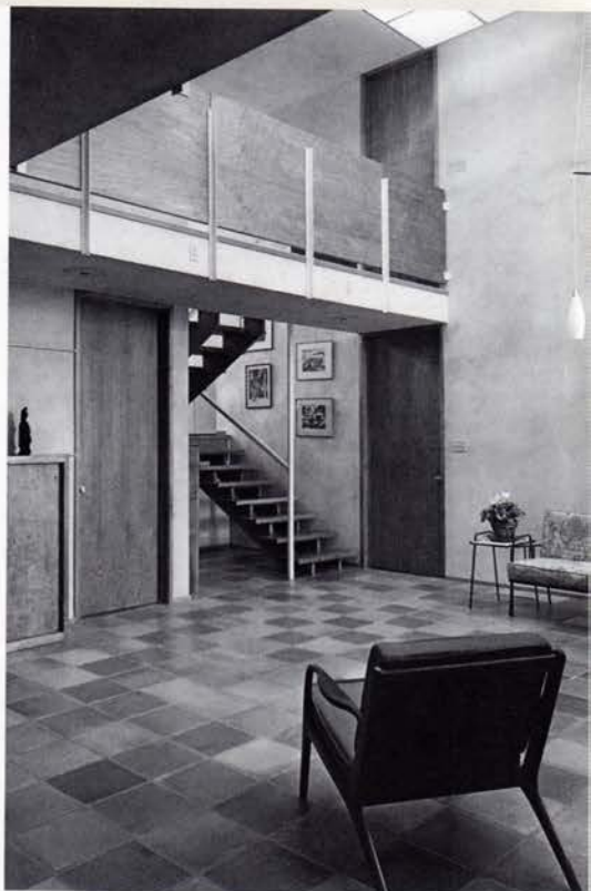
The home's signature space, a 20-foot-square interior court, is far from ostentatious. The upper-level guardrails, for example, are repurposed hollow-core wood doors.
