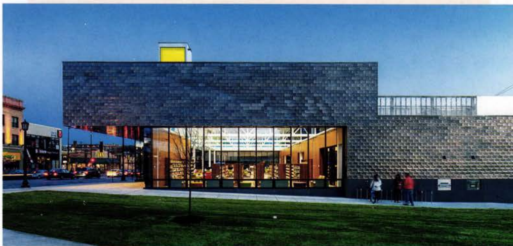
Top: The intimately scaled children's area features bright colors and large letters on the ceiling. Above: VJAA used a durable and cost-effective roofing system of stainless steel panels for exterior cladding.
