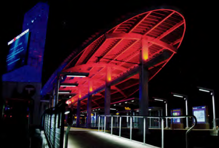
Target Field Station - Minneapolis
