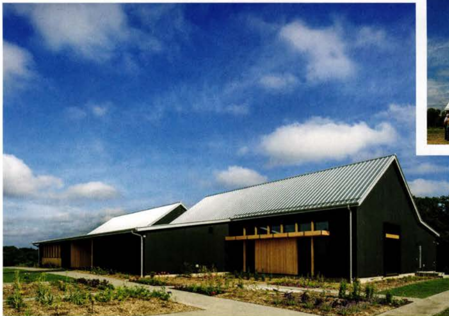
A lower roof over the entry breaks down the scale of the long building. The shed roofs echo the agricultural vernacular of the existing Red Barn. The charcoal-colored wood is Accoya, an extremely durable heat-treated wood.
