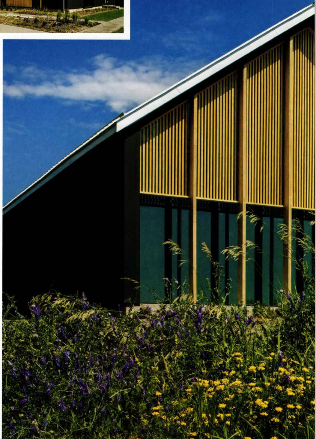
A lower roof over the entry breaks down the scale of the long building. The shed roofs echo the agricultural vernacular of the existing Red Barn. The charcoal-colored wood is Accoya, an extremely durable heat-treated wood.
