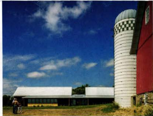
A lower roof over the entry breaks down the scale of the long building. The shed roofs echo the agricultural vernacular of the existing Red Barn. The charcoal-colored wood is Accoya, an extremely durable heat-treated wood.
