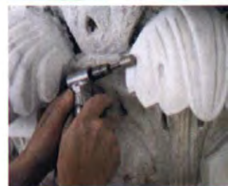
One of the many stonemasons on the project blends a Dutchman replacement into one of the building's many capitals.
