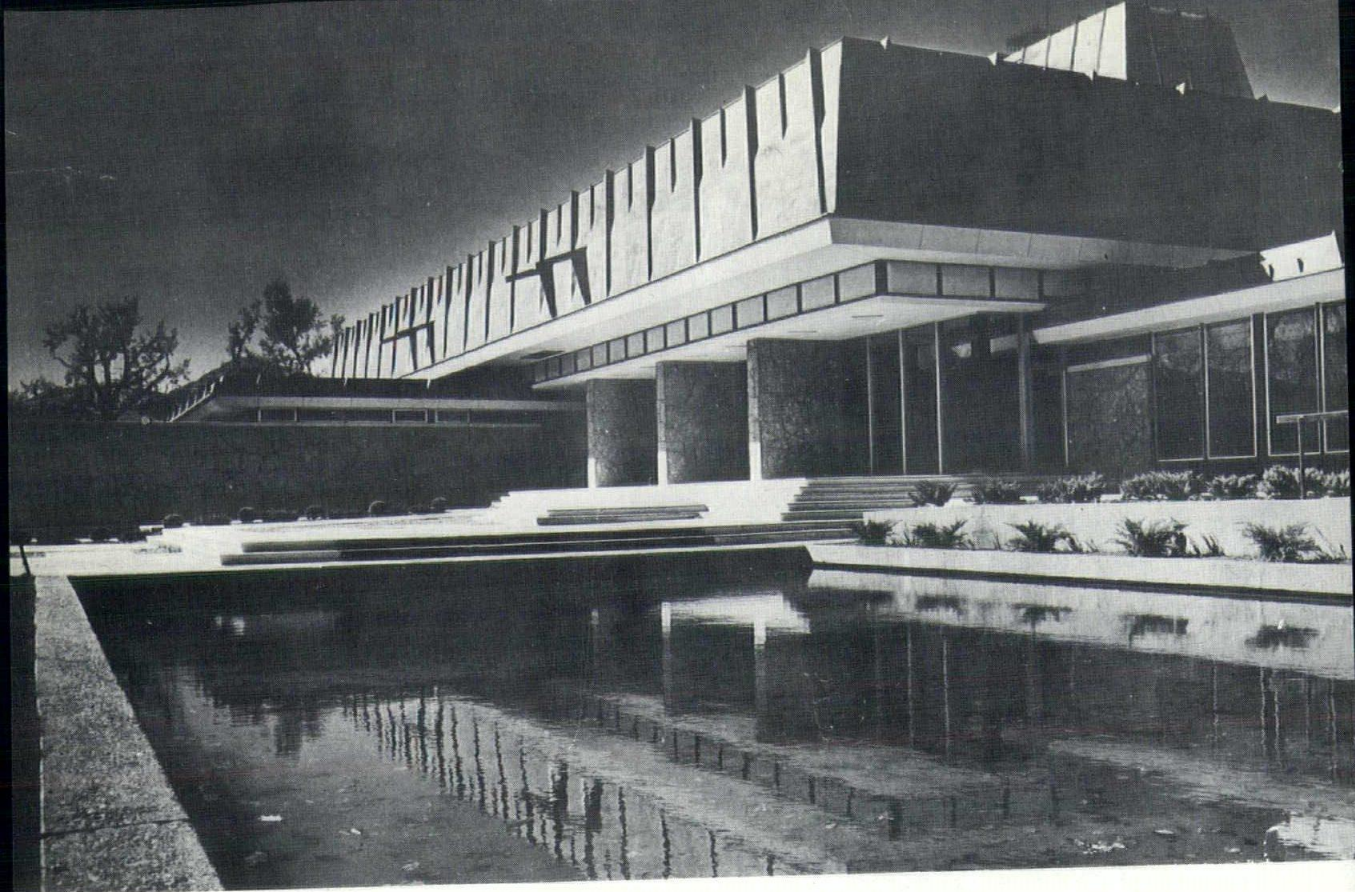
Thirty-five thousand pounds of 16-ounce sheet copper was supplied by Chase Brass & Copper Co., for the new $1.2 million Fremont County Court House shown here. A total of 32 panels of copper, 16 feet long by 11 feet high by four-inches-thick, were laminated to rough-surfaced native marble for the exterior walls. Each panel weighs 5,000 pounds.
