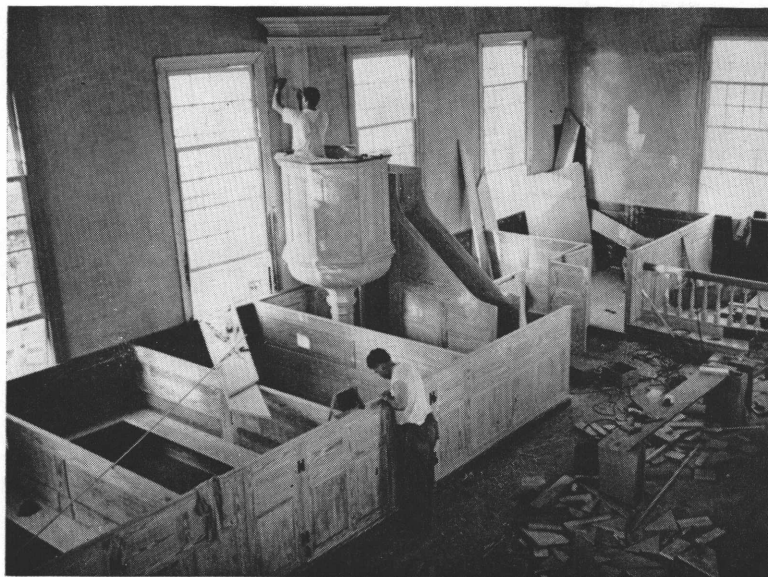
Replacement of interior furnishings is being accomplished in this view, which is one of the several hundred made to record every research procedure and the techniques employed in the restoration of St. John's Church.
