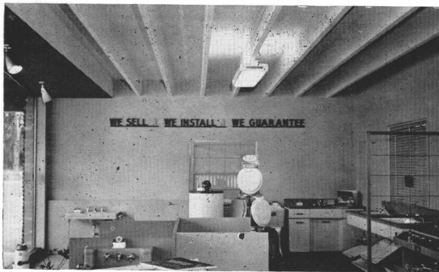
Commercial building with double tee roof units 40 feet clear span on load bearing exterior walls.
