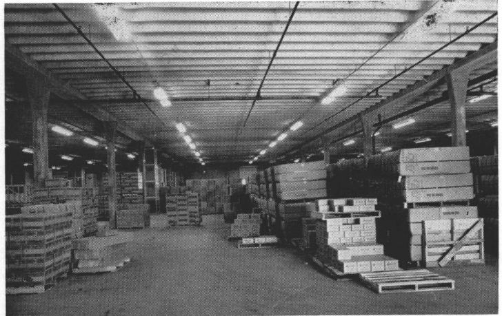
above: Precast, prestressed columns, girders and double tees in typical 25' x 40' bays.
