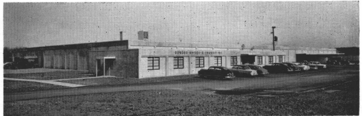
below: Exterior walls of Tilt-up concrete construction. Panel size: 16' x 20' x 5".
