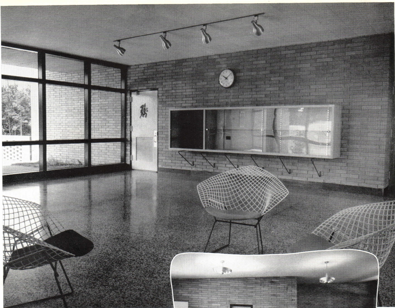
Shamrock Garden Elementary School Charlotte, N. C. (City School) Architect—Edwin Wilson Load Bearing 10" all brick cavity walls
