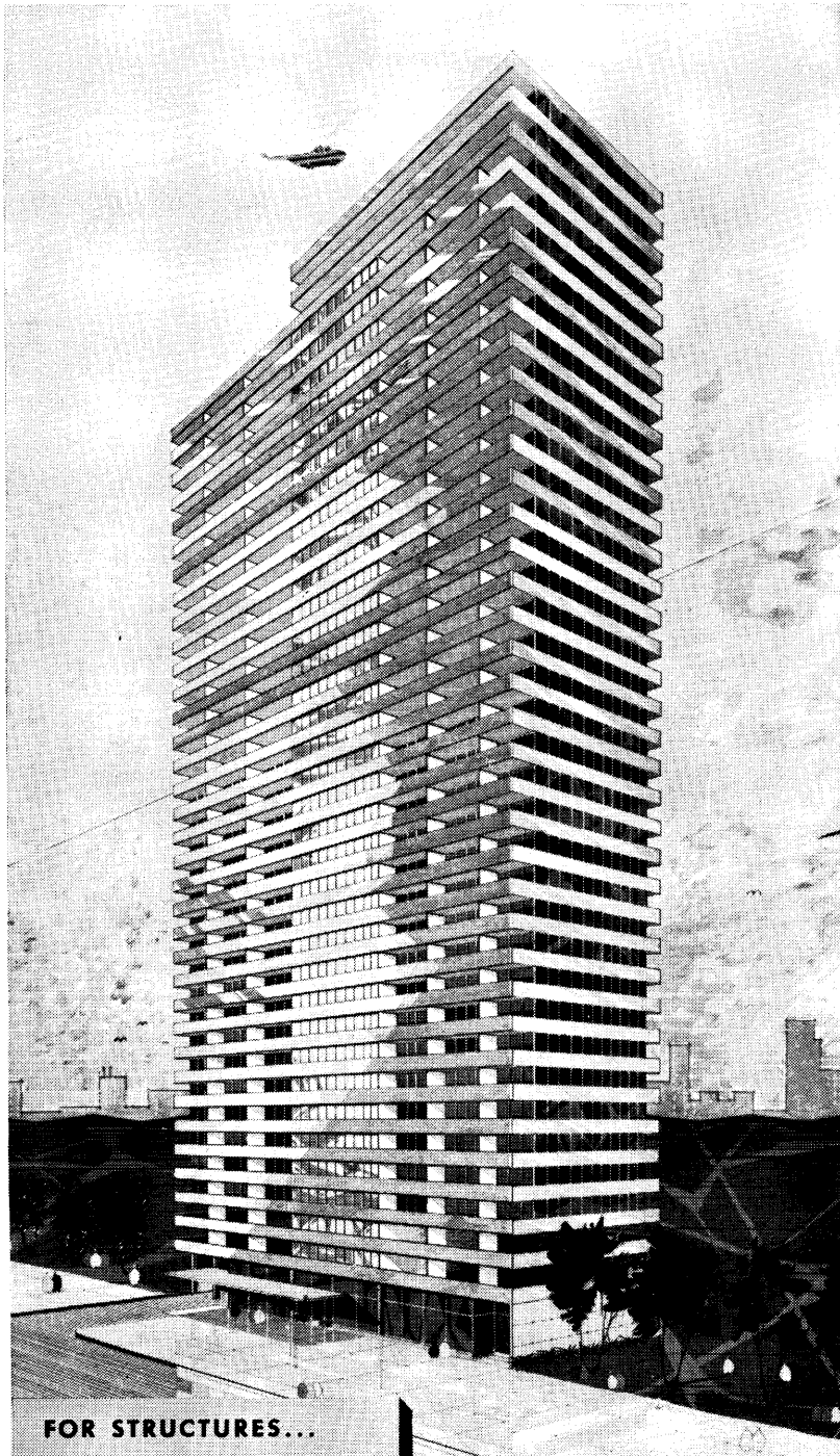
Four concrete shear walls extending across the width of the building provide necessary resistance to wind forces.
