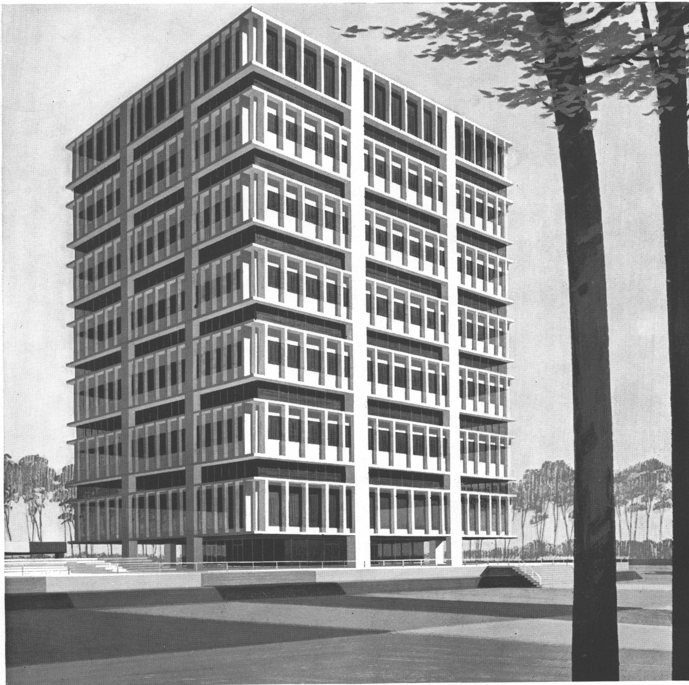
The nation's tallest precast, post-tensioned concrete building, headquarters for the North Carolina Mutual Life Insurance Co. in Durham, has exposed concrete columns and trusses. Architect: Welton Becket & Associates, Los Angeles.
