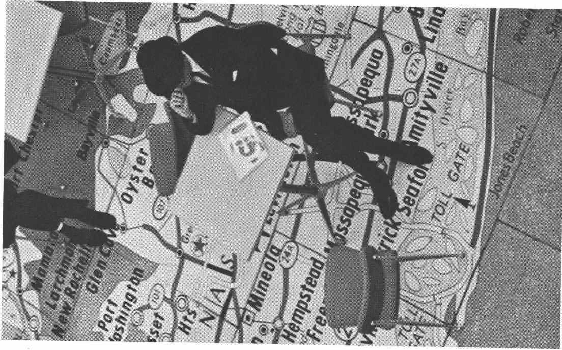
In the floor of the New York State Pavilion at the New York World's Fair, multi-colored terrazzo ingeniously traced the outlines of the major highways across the state. Architect: Philip Johnson Associates, New York. Terrazzo Contractor: Port Morris Tile & Terrazzo Corp., N.Y.
