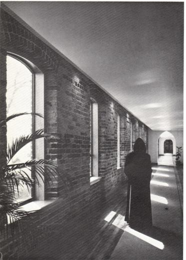
When work began on renovating the 1881 monastery at Belmont, the building was in both good and bad shape. With its 18 inch thick, load bearing brick walls and its heavy timber construction, it was in good enough shape to save. (The cost of replacing it, put at \$4 million, was prohibitive, anyway. The final cost of renovation came to only \$878,000.) But even while the architects were analyzing the building before beginning to design, one of the ceilings fell. Clearly, something had to be done.
