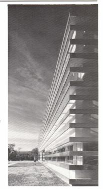
Though designed, constructed and occupied in a total elapsed time of only seven months, the Southern Service Center of the Equitable Life Assurance Society avoids the tried and true solutions of the speculative office building. On the contrary. This building not only has a carefully detailed aesthetic, but it incorporates some fancy innovation—a new way to use the sun to warm the building in the winter and to use cooled air to insulate in the summer.
