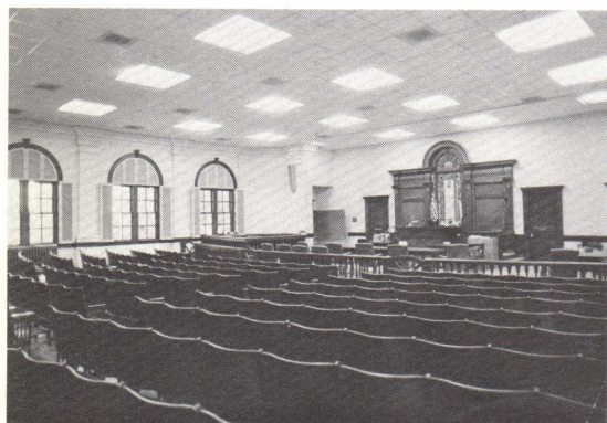
Left: Anson County: Lowered ceilings are detrimental both aesthetically and acoustically
