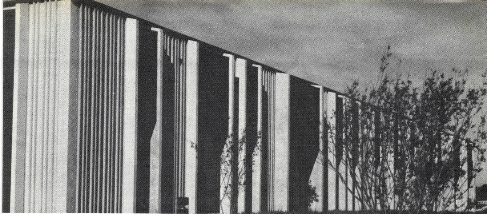
Deep Rib Corewall Panels — Allen Bradley building, Greensboro Architect: John D. Latimer, AIA. Contractor: JMD Contractors
