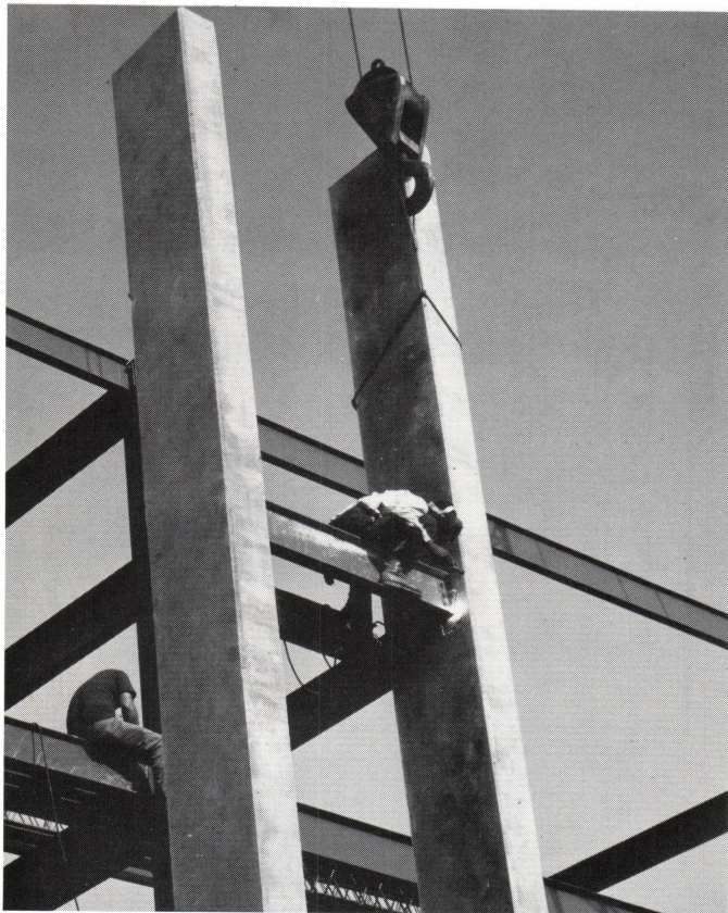
(Right) Erection of 18 ton end panels (Below) Site erection technique
