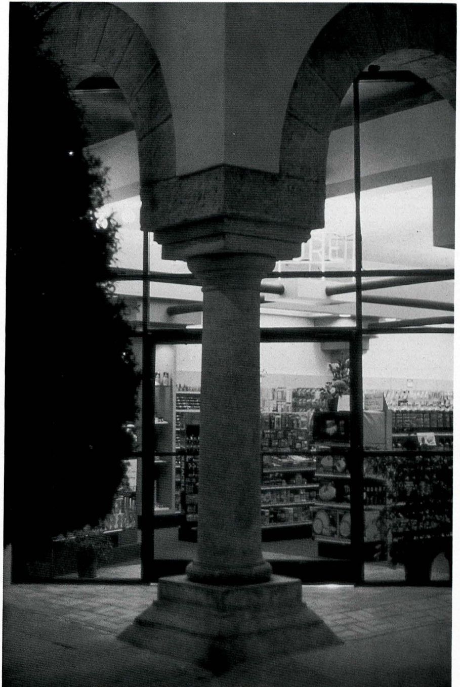
Granite columns and arches, covered with masonry and stucco during the 1950s, were exposed in the restoration.
