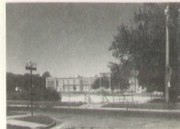
Figure 8—Northeast playground entrance and rear view of school building.
