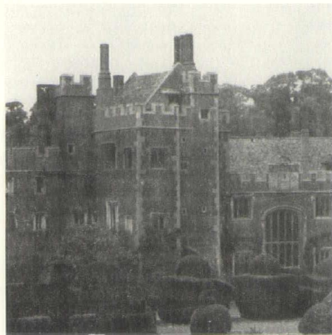
4. View from southwest
