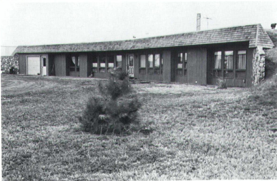
View of the house from the south. November 1983
