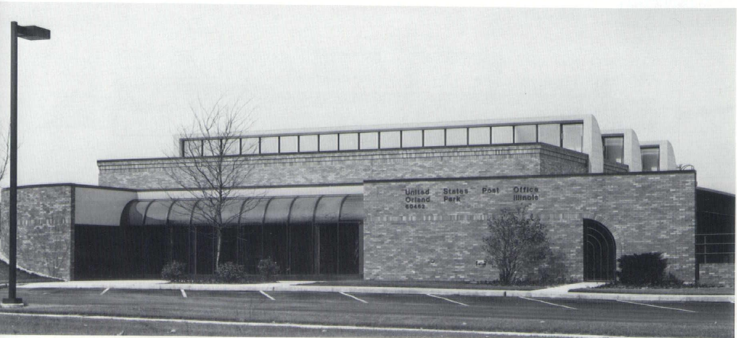
South view of the post office showing sky scoop monitors with clear glazing for maximum heat intake.
