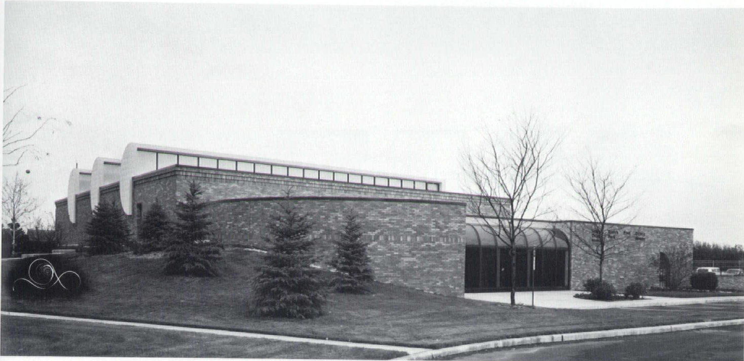
Southwest view of the passive solar post office showing berming on the building's western exposure.
